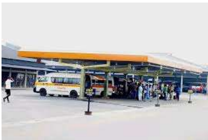
Figure 1. AKTC Park Terminal, Uyo
