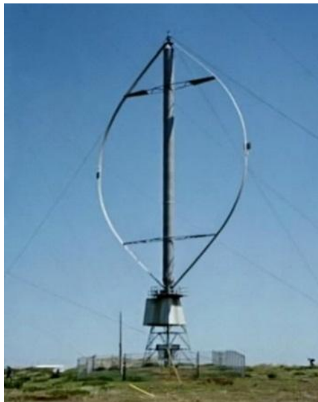
Figure 5. Darrieus Wind Turbine
