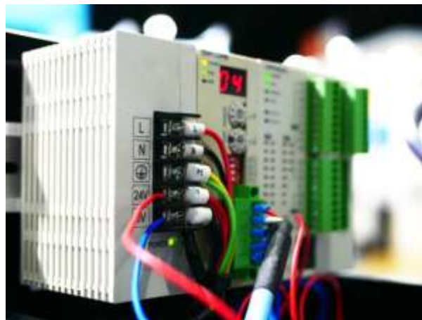
When self-starting generator is starting
